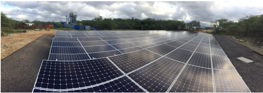
A newly installed 134 kW photovoltaic array at Joint Base Pearl Harbor Hickam, Hawaii, is part of the Pacific Energy Assurance and Resiliency Laboratory, a renewable energy microgrid project demonstrating new ways for military facilities to address energy needs. (Photo courtesy of HNU Energy/Joseph Cannon)
